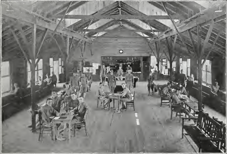
FIG. 52.—Interior of Young Men's Christian Association hut.
